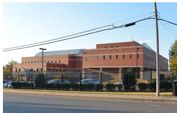
View of South Facade
