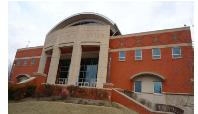
Public Entrance to security screening
