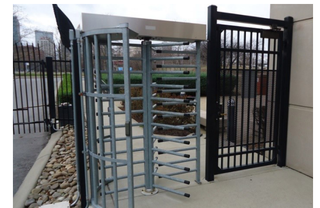
Secure parking lot turnstile
