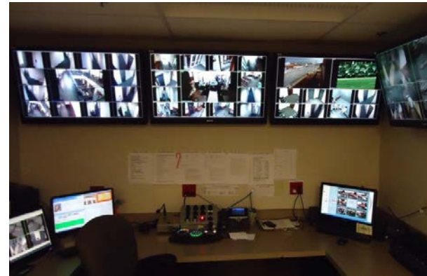
Security Control Room
