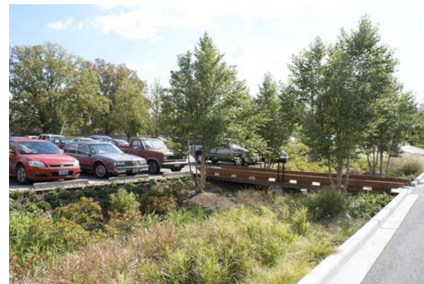
Bioretention devices can retain stormwater until it infiltrates, allow for native species planting and habitat restoration, and provide visual interest for relaxation and recreation.
