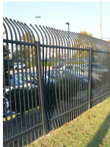
No climb fence
