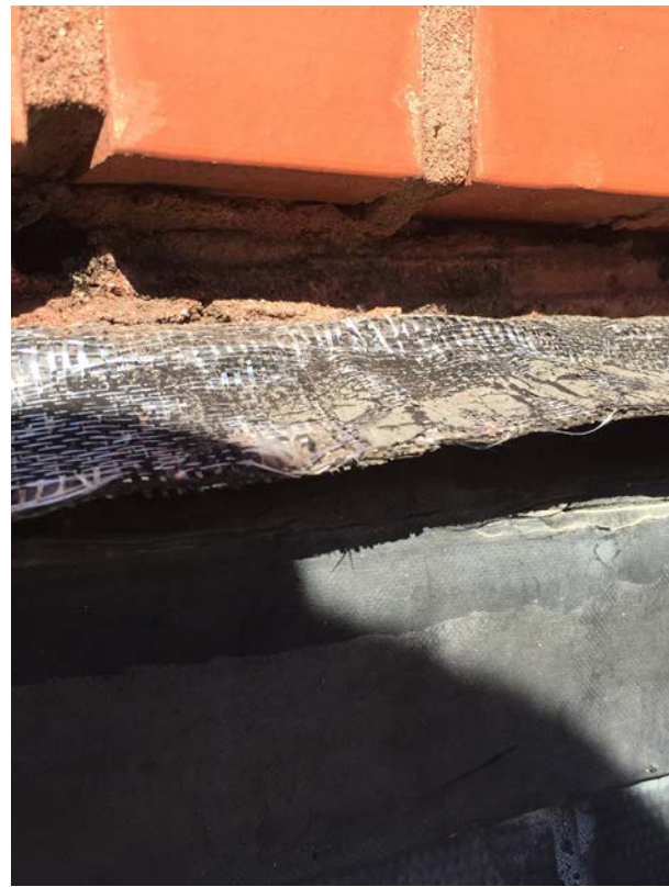
Through-wall flashing
