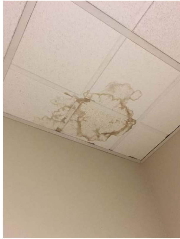
Water damage at ceiling tile
