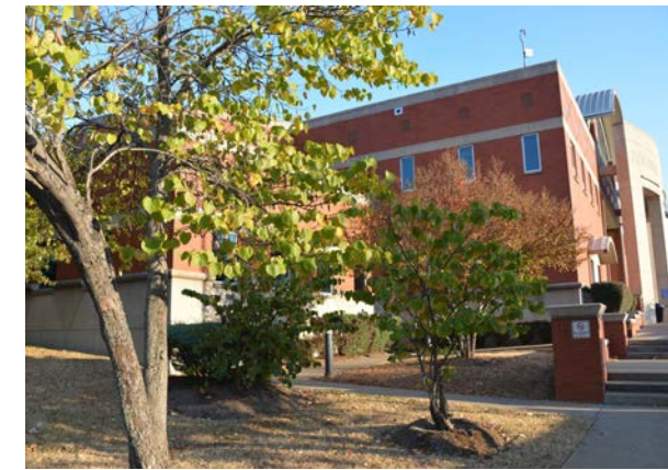
Sidewalk /Ramp (Northwest Side)
