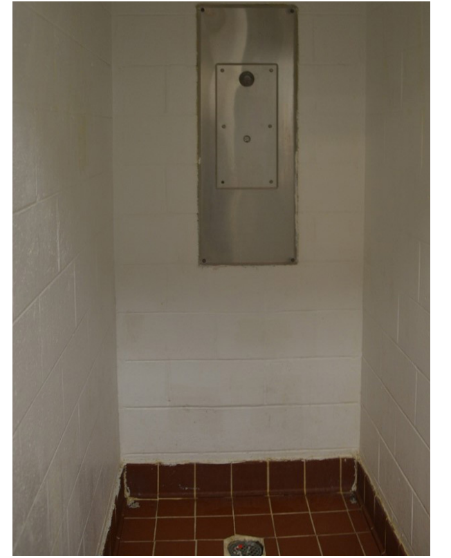
Damaged floor tile
