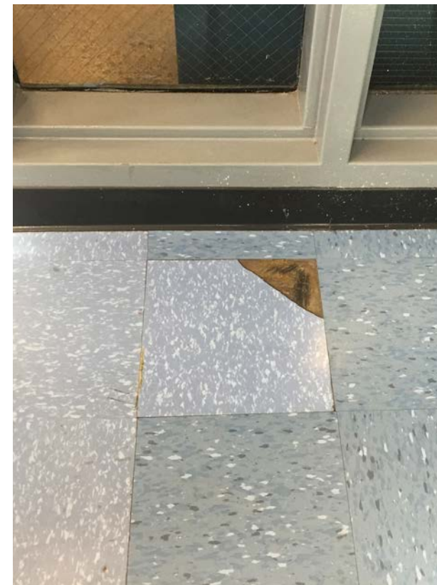
Floor at Detention Area
