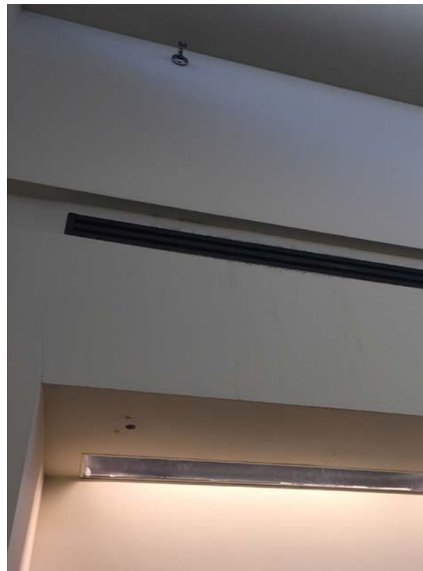
Damage at ceiling tile
