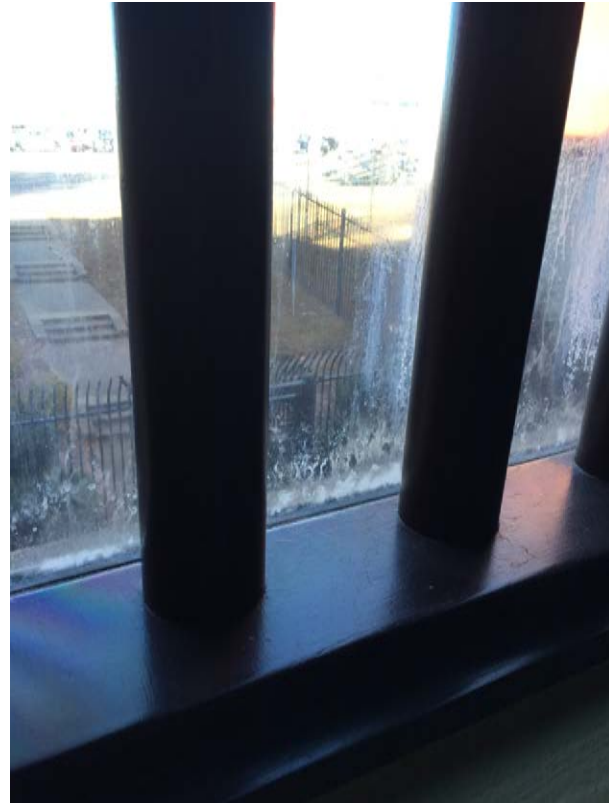
Window leakage
