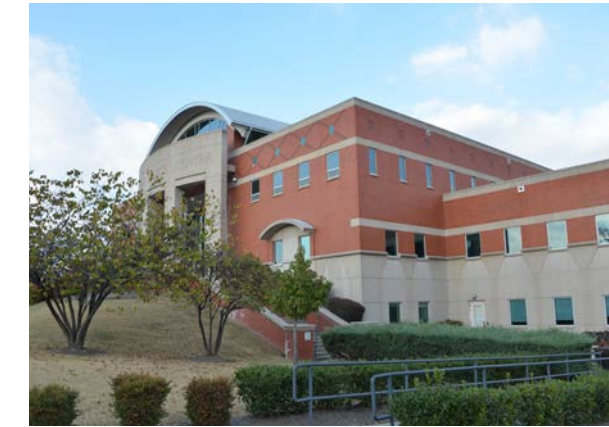
View of Southwest Facade
